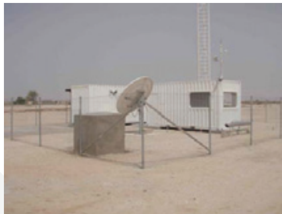
The Mauritania radionuclide monitoring station installation
